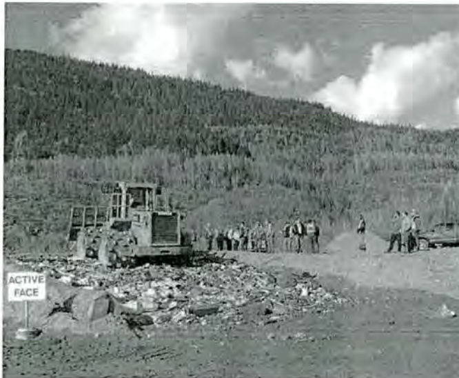
Figure 5-3: A Well-Defined Active Face of a Landfill Cell
