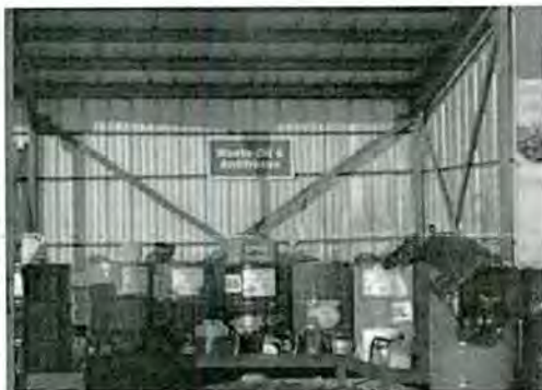
Figure 6-1: Sheltered Receiving Area
